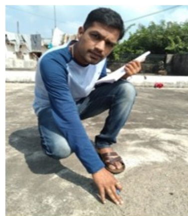
Figure 4: Selected Roof for insulation
